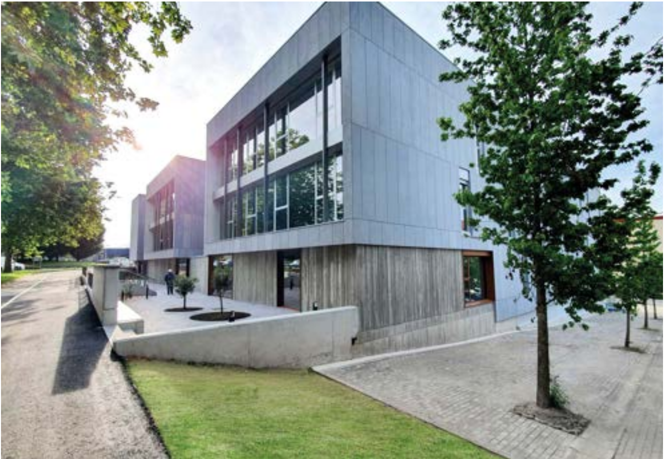
Cofinimmo decided to pursue a new path, which ultimately led to it becoming a juggernaut in the European healthcare space (here a nursing & care home in Oleiros, Spain, with BREEAM Excellent certification).
