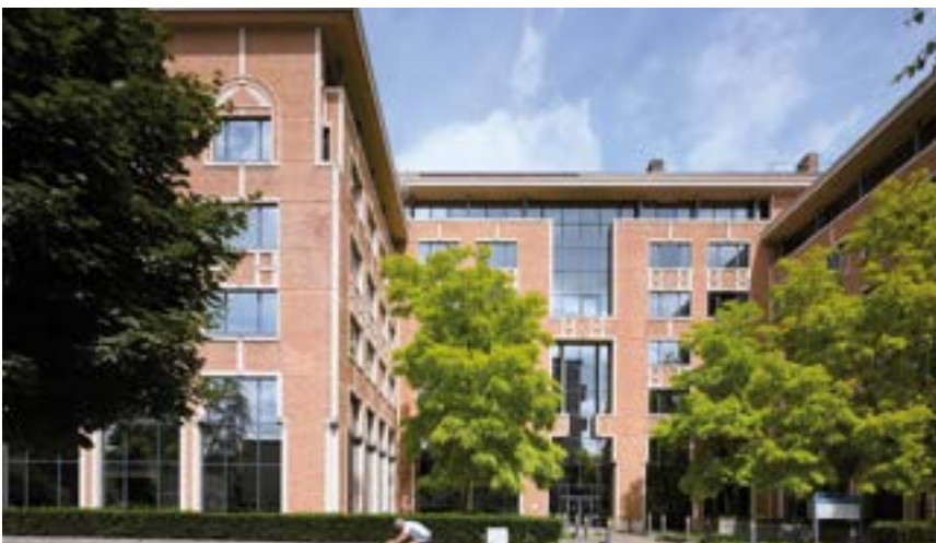
Antares is a project completed in 2021. Inclusio renovated an old office building in 79 affordable housing apartments in Woluwe St Lambert (Brussels).
