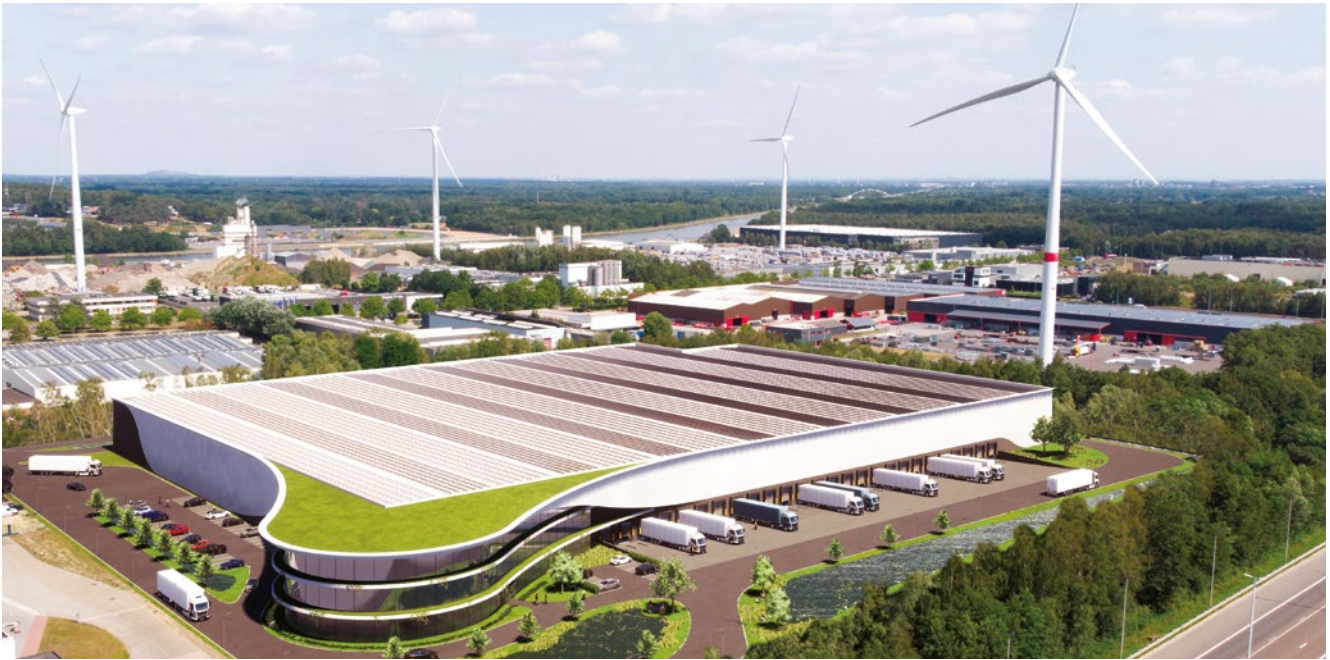
“Lummen Carbon free” - Montea’s project of the first carbon-free building for logistical activities in Belgium
