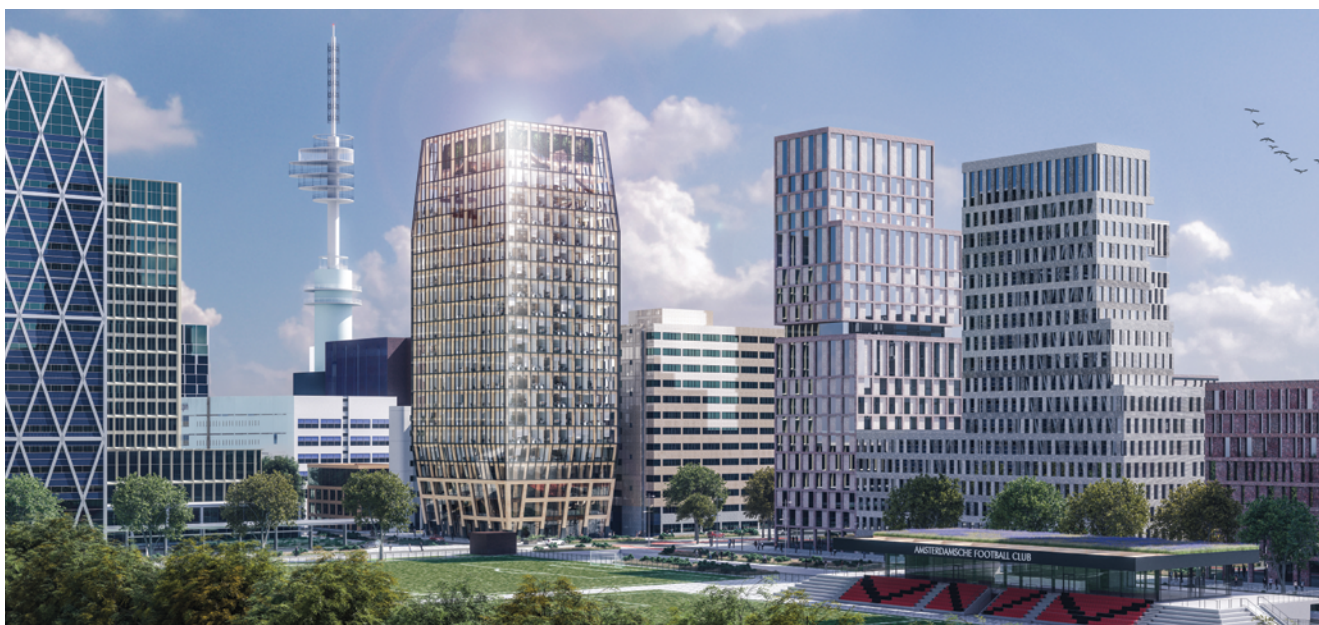
New wooden office building
