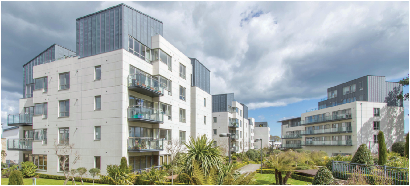
Irish Residential's Beechwood Court, Dublin
