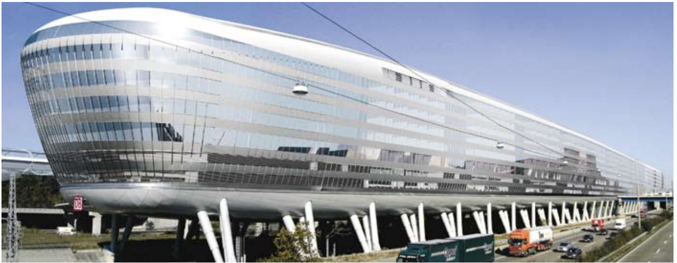
Airrail project at Frankfurt's Rhein-Main Airport.
